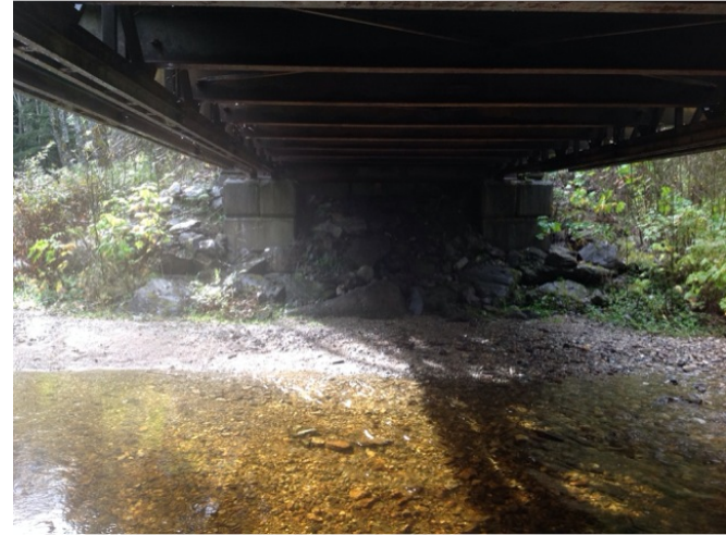
Left Bank Abutment when facing downstream
