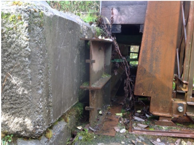
typical ballast wall
